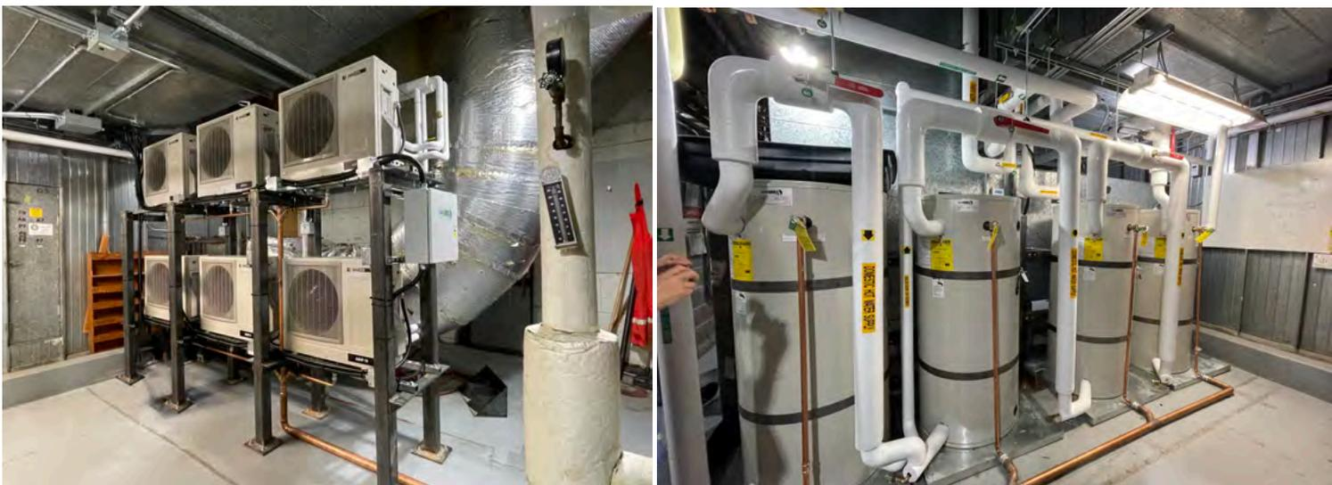
Installed system shown with 6 x Heat Pumps, 4 x SAN-119 gallon tanks and the SANCO<sub>2</sub> Controller for the system
